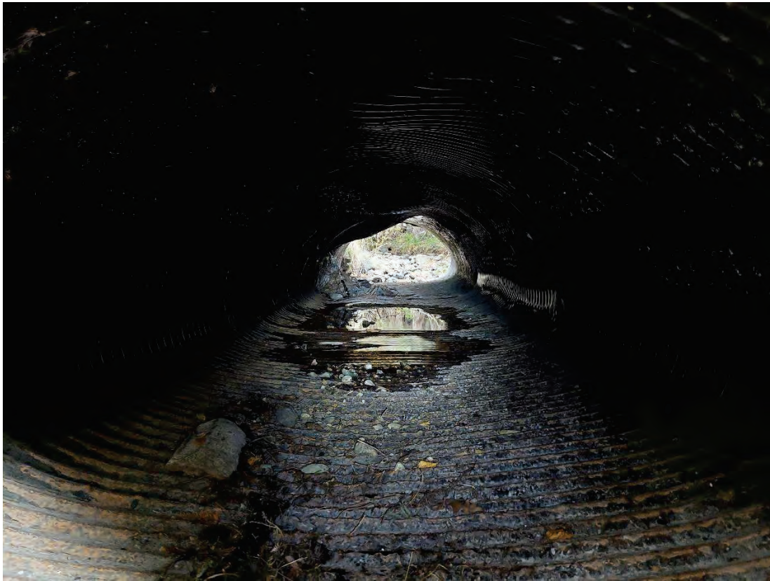
Culvert Inlet facing US: Buckling visible at multiple locations, flow disappearing at pipe invert
