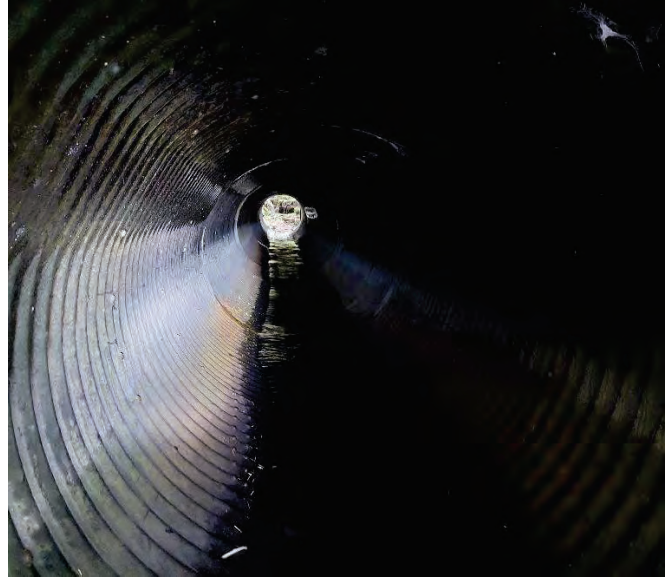
CULVERT 14 (3442927) INTERIOR: MINOR PIPE SEPARATION
