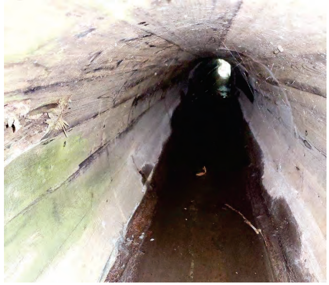
AREA 2 MARBLE RD: WOOD STAVE CULVERT (3442931) INTERIOR
