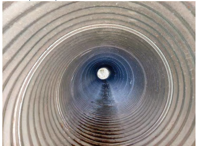
CULVERT 11 (2254788) INTERIOR: GOOD PIPE CONDITION
