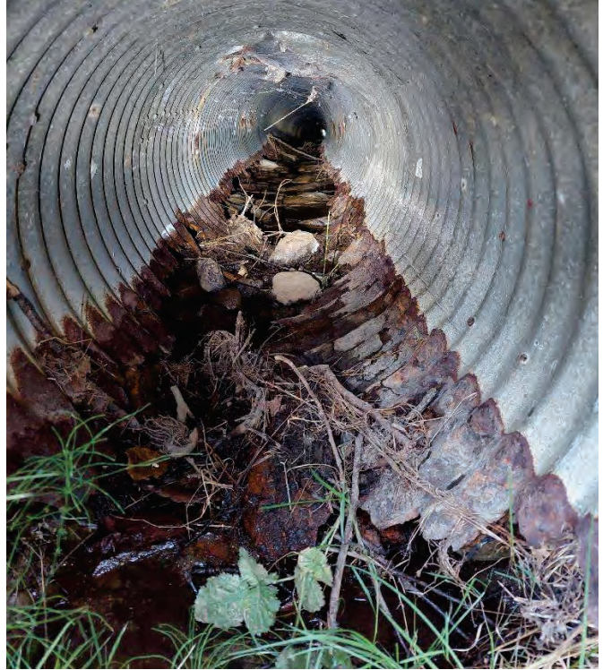
AREA 4 SANDERSON RD: CULVERT (2258625) PIPE INVERT CORRODED AWAY LOOKING DOWNSTREAM
