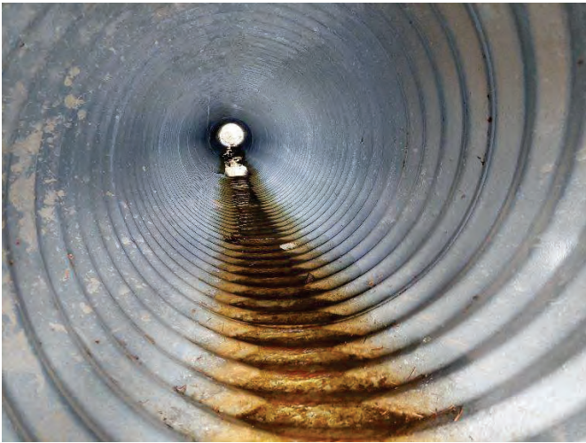
AREA 4 GILLIES BAY RD: TWIN 600MM CSP CULVERT INLET AT TENNIS COURT
