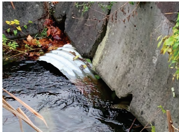
PHOTO 2: AREA 1- FULL FLOW (VID, NOVEMBER 2023)
