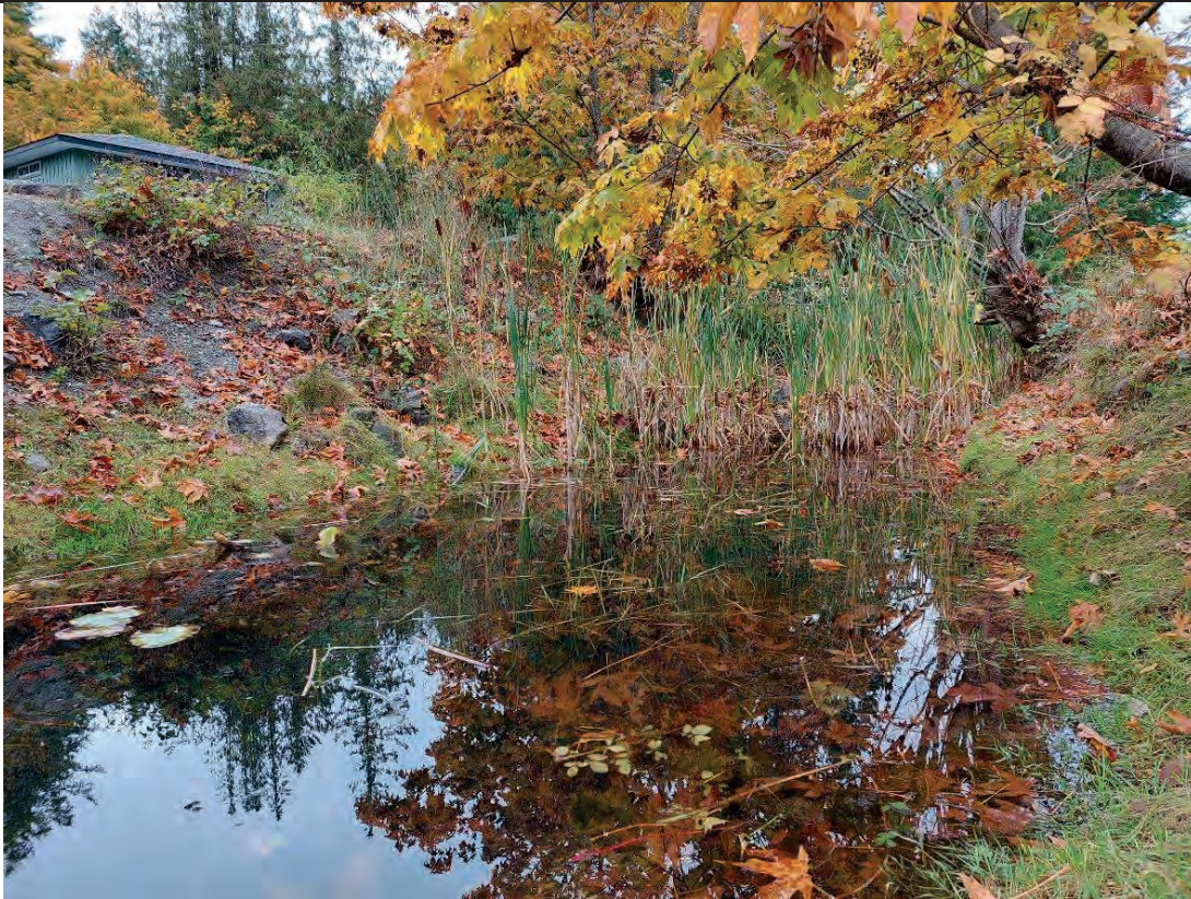
Upstream Channel facing US: Bank erosion visible on the left side
