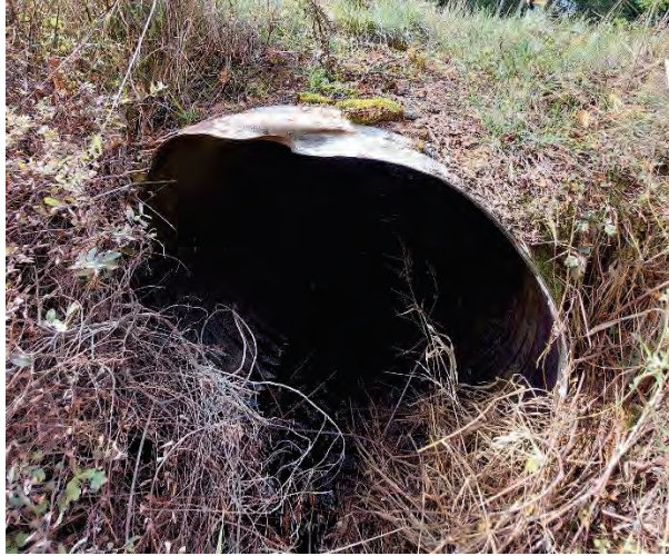
CULVERT 12 (2255061) INLET: INLET BEND
