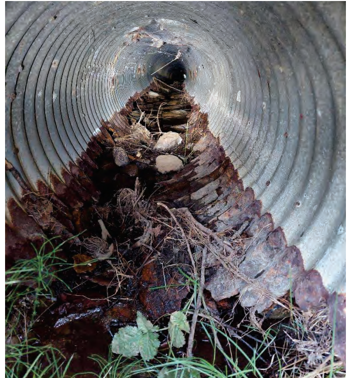
CULVERT 6 (2256019) INTERIOR: PIPE JOINT SEPARATION AND ROCK DEBRIS
