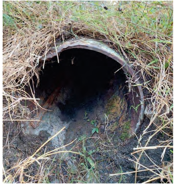
AREA 4 AIRPORT RD: 300MM CSP CULVERT (2258675), HEAVILY CORRODED INVERT
