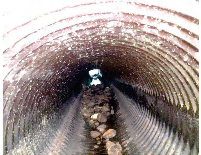
CULVERT 6 (2256019) INTERIOR: PIPE JOINT SEPARATION AND ROCK DEBRIS
