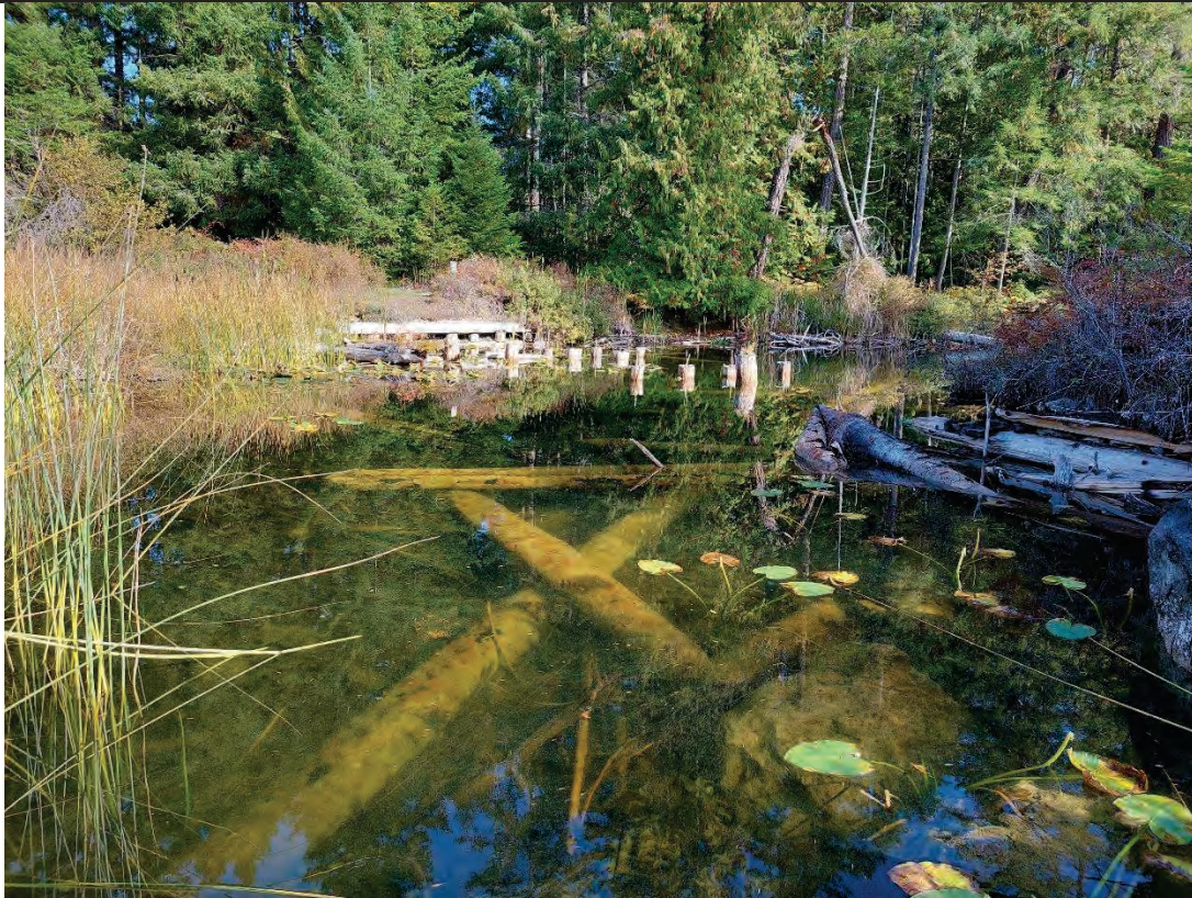
Downstream Channel facing DS: Woody debris and old CSP pipe visible, sensitive habitat for painted turtle
