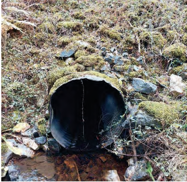
CULVERT 14 (3442927) INLET: PIPE COATING INTACT
