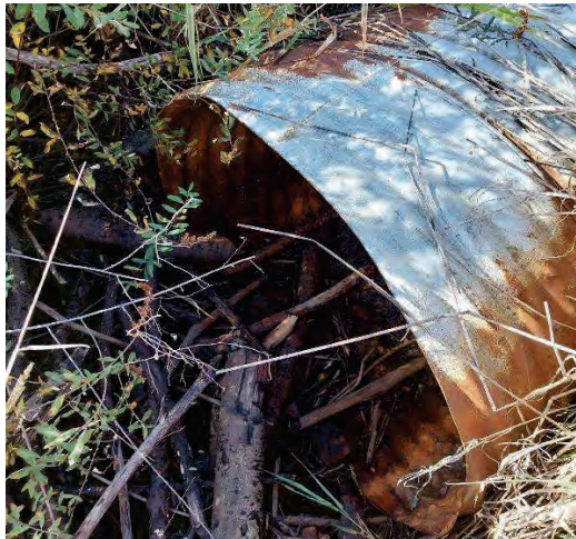
CULVERT 4 (2256045) INLET: MINOR WOODY DEBRIS
