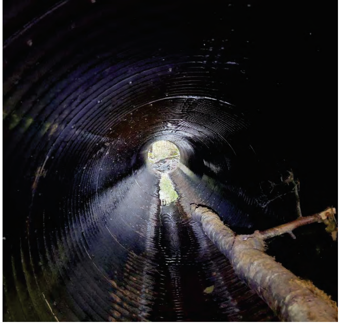
CULVERT 9 (2256424) INTERIOR: PIPE COATING MOSTLY INTACT
