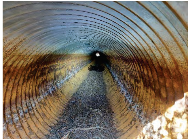
CULVERT 1 (2254949) INTERIOR: MATERIAL CHANGE AND HEAVY CORROSION
