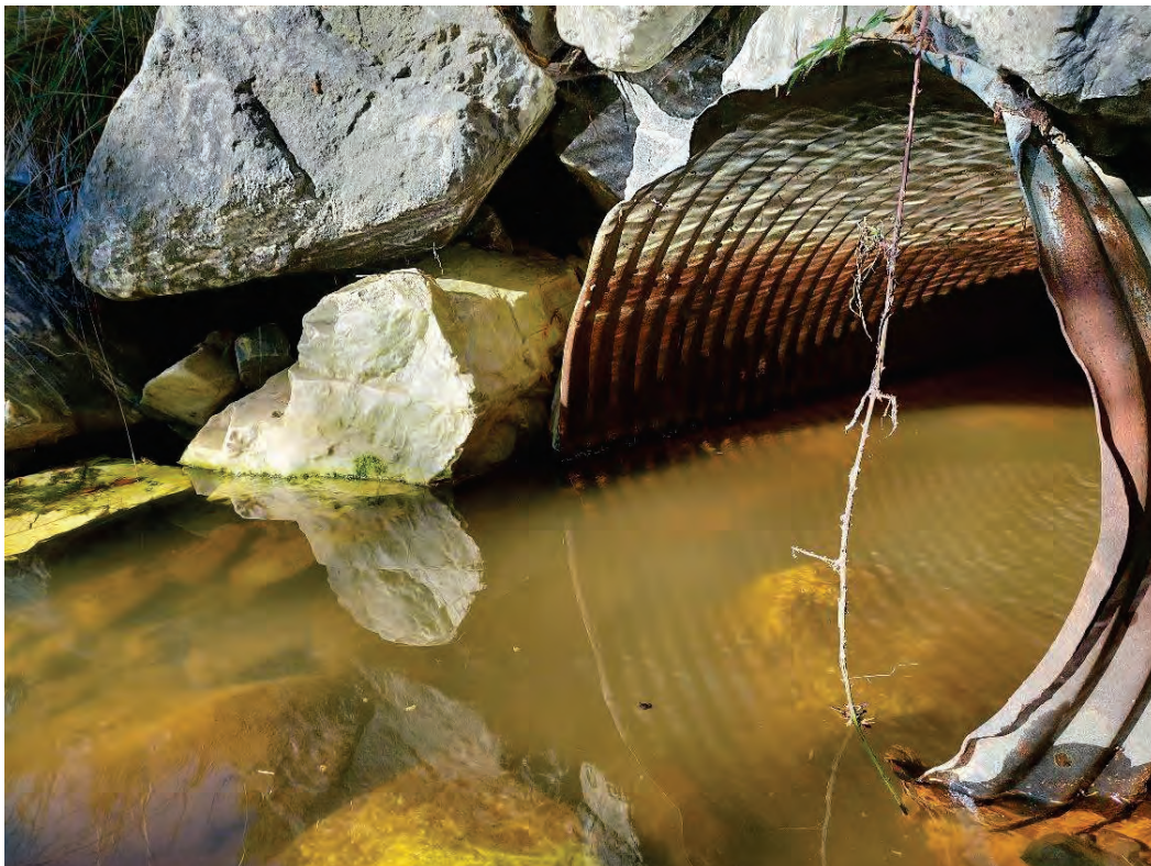
Culvert Outlet: 1200mm CSP pipe with riprap headwall
