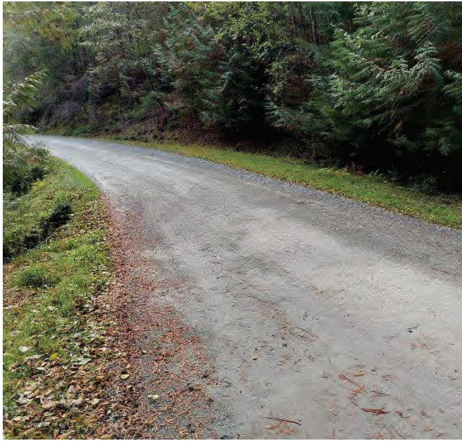
CULVERT 13 (3442926) ROAD: CENTRAL ROAD ABOVE CULVERT
