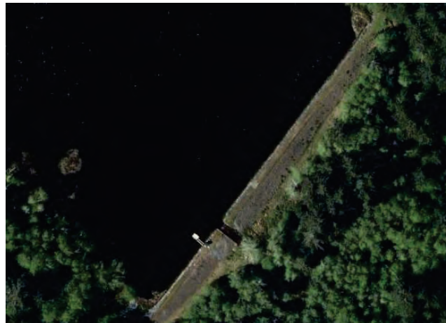
PHOTO 7: ORTHOGRAPHIC IMAGE OF CRANBY LAKE DAM AND SPILLWAY (ESRI)
