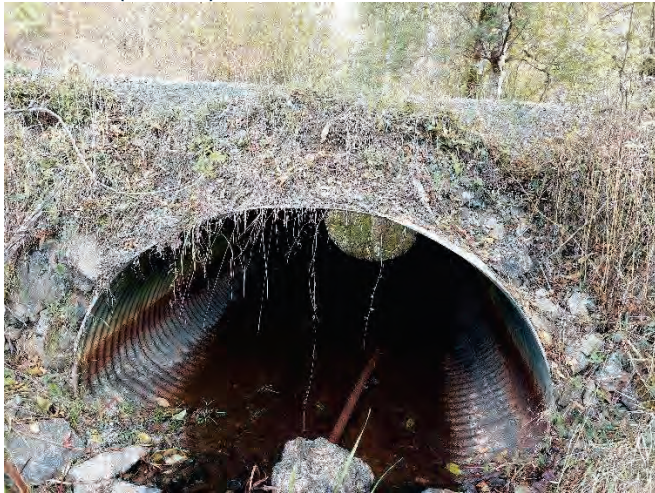
CULVERT 14 (3442927) INLET: PIPE COATING INTACT
