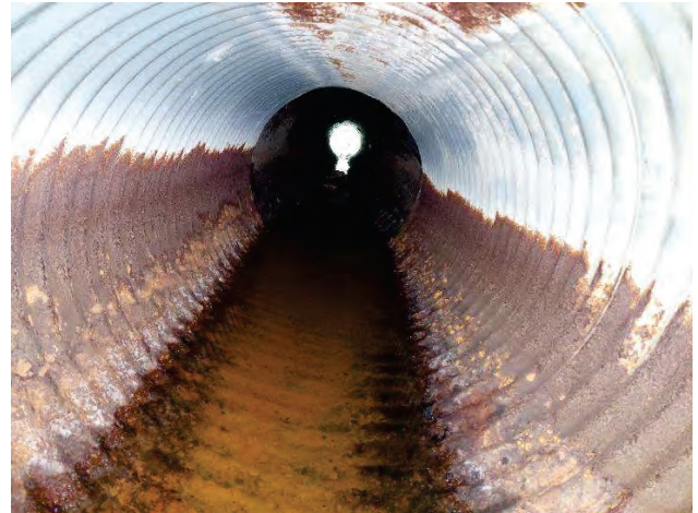
CULVERT 1 (2254949) INTERIOR: MATERIAL CHANGE AND HEAVY CORROSION
