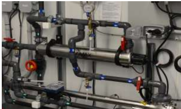
Figure 2.8 Housing for activated carbon cartridges
