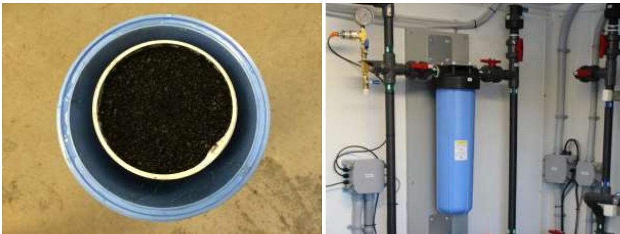
Figure 2.7 Refillable granular activated carbon cartridge (Left) & housing for activated carbon cartridge (Right)
