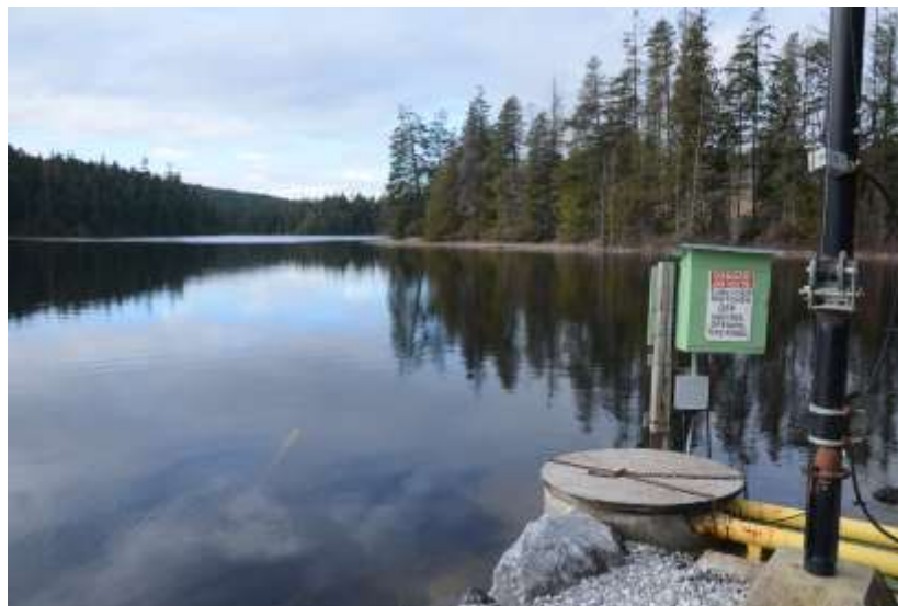
Figure 1.2 Water is gravity fed in to a well and pumped to VAID's water treatment system
