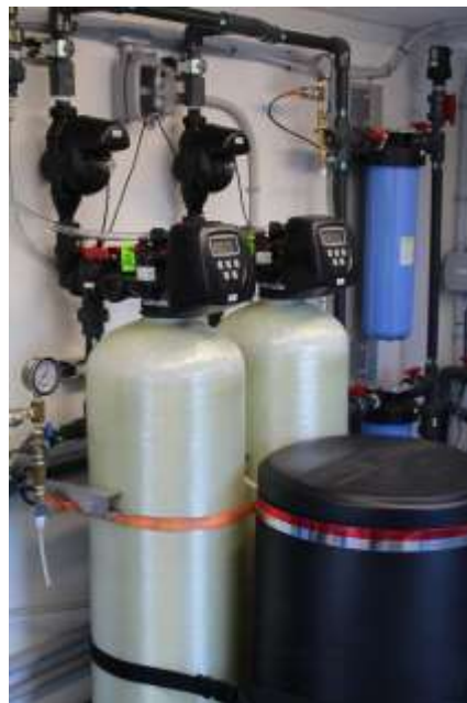
Figure 2.6 Ion exchange reactor where the raw water is mixed with the resin
